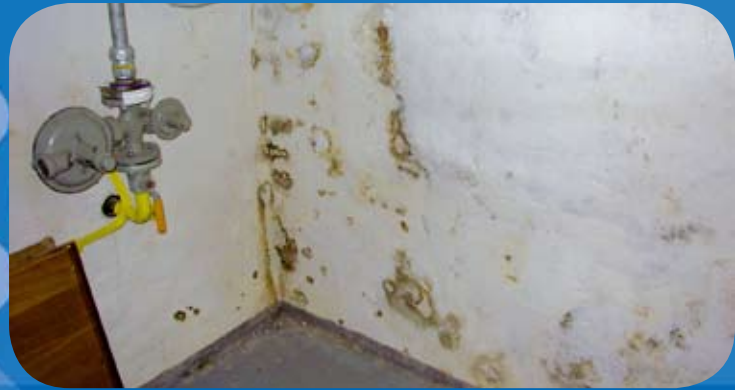
Wet walls can cause extreme damage such as a proliferation of mold.
